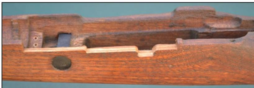
As with all side mounts, wood has to be removed to accommodate the base and this should be done after the bedding, therefore guaranteeing a consistent fit. As the reader may note in the 2<sup>nd</sup> picture, failure to remove metal from the underneath of the base results in more wood having to be removed from the stock, which in turn will result in a unsupported recoil bolt.
