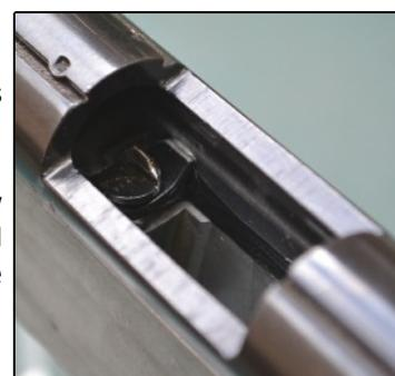
The receiver has a typical rimfire dovetail for mounting a scope with two pairs of punch marks as can be seen on the picture. They are machined punched, so they have not been applied at a later date. Therefore I assume they are some form recoil stop for the scope rings but I can't see them as serving any real purpose.
